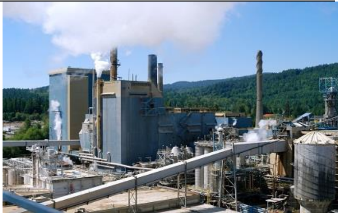
Crofton Mill, Power and Recovery Area
