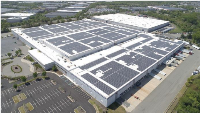
Figure 1: IMDC 7.2 MW solar installation, Edison, NJ
